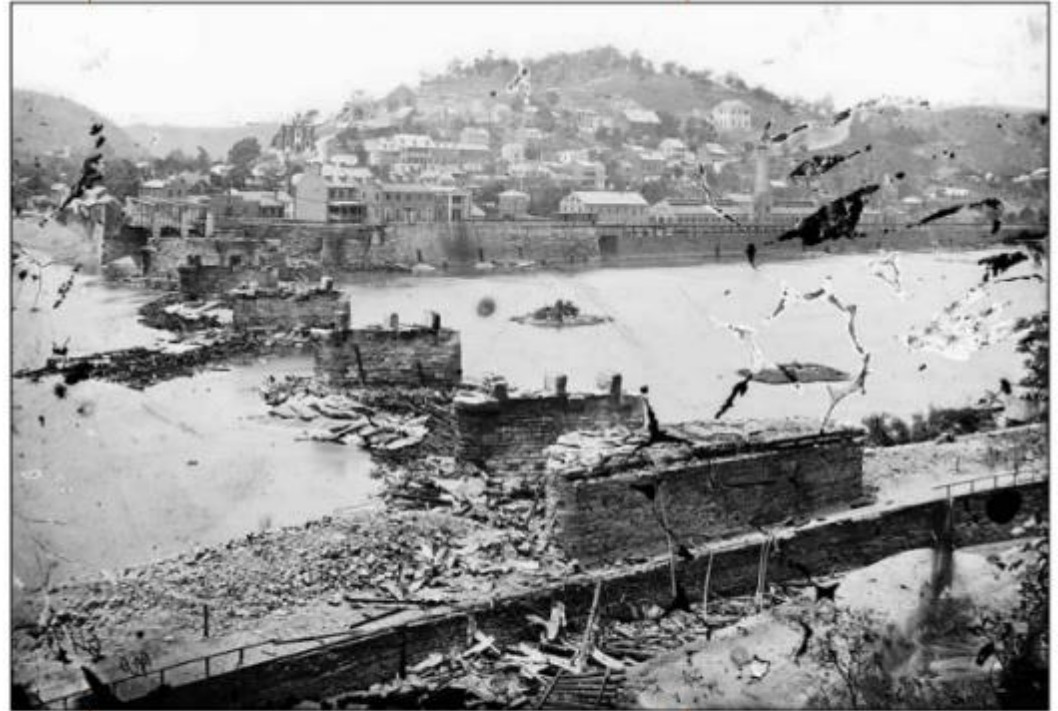
Ruins of the B&O Railroad bridge at Harpers Ferry, June 1861. (Library of Congress)
